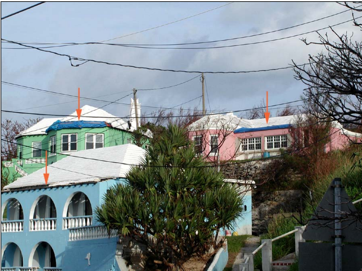
Figure 2. Widespread "leading-edge" roof damage on south facing Mullet Bay Road, St George's.
