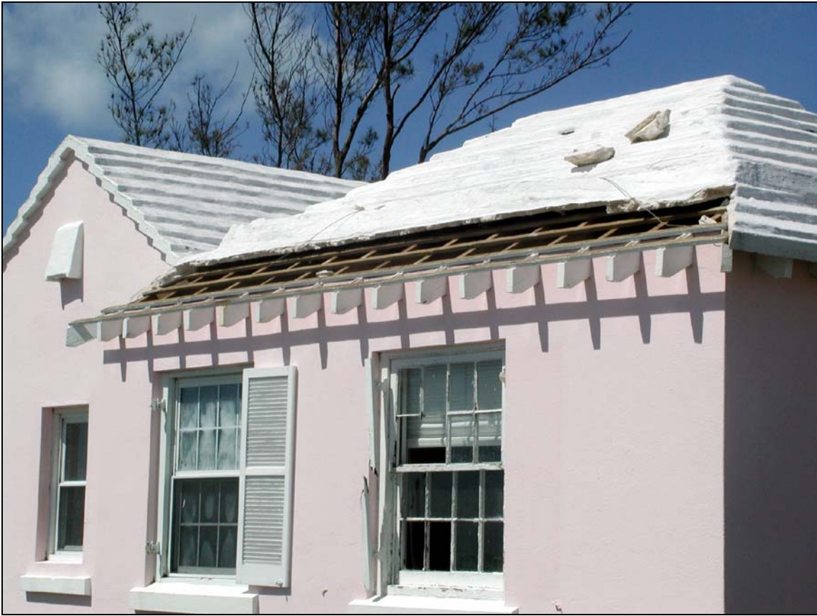
Figure 3. Typical leading-edge damage. Berry Hill Road, Devonshire (south facing).
