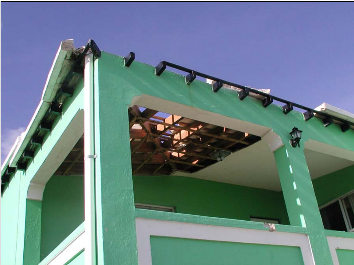
Figure 12. Verandah damage, Knapton Hill, Smith's Parish (south facing).
