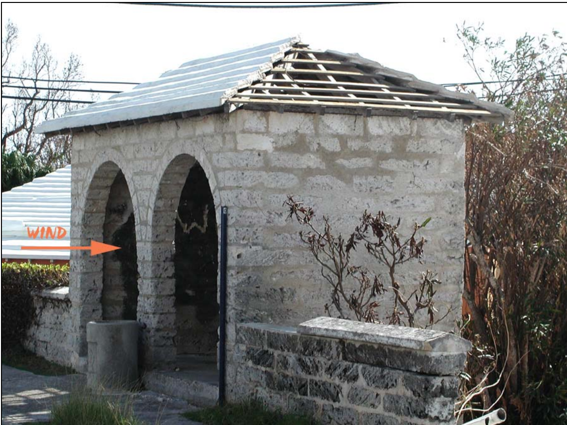
Figure 10. Rare leeward side damage. Due to pressurization within open structure. (north facing).
