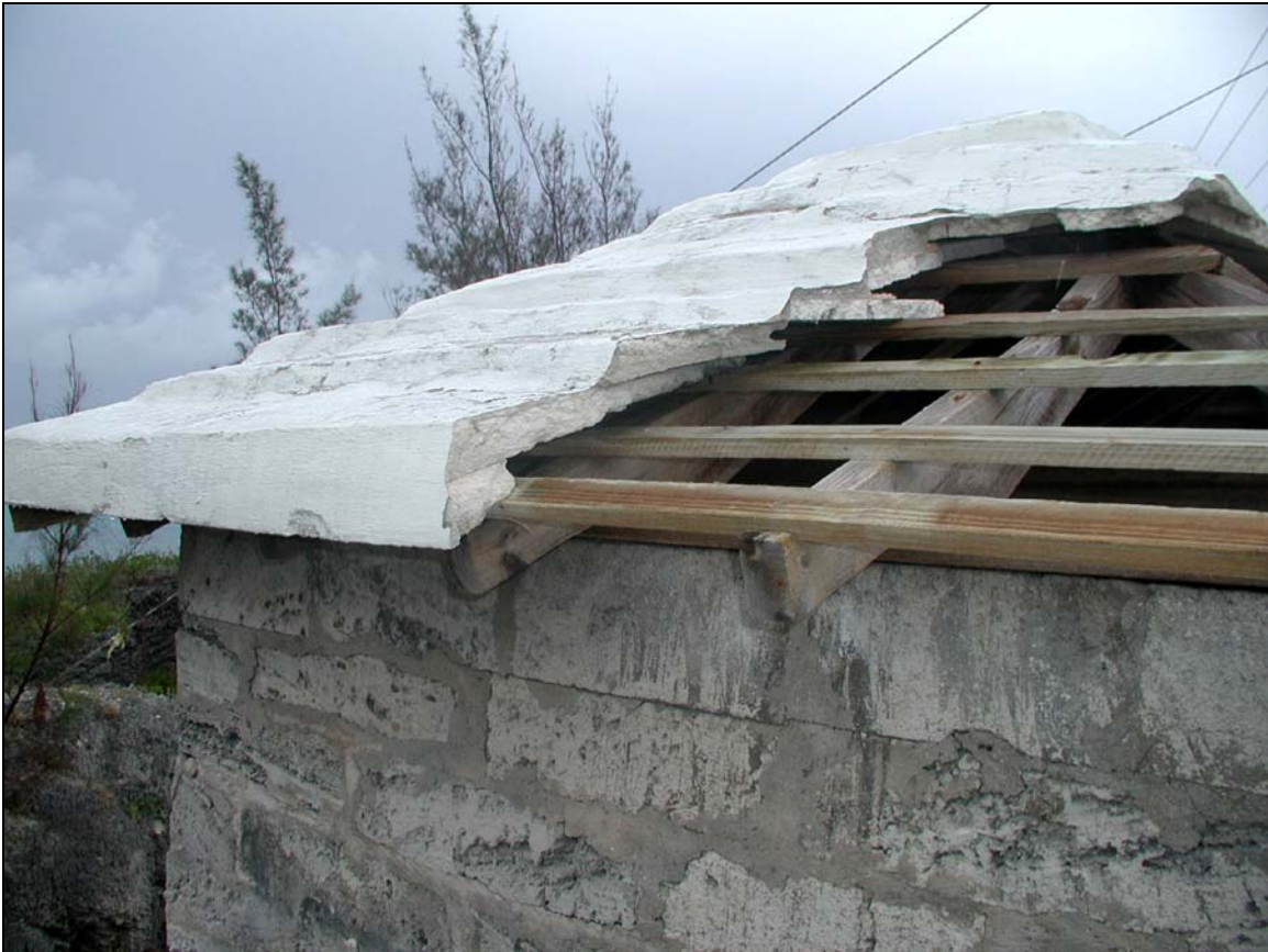
Figure 45. Damage reveals construction details of a traditional limestone slate Bermuda Roof.
