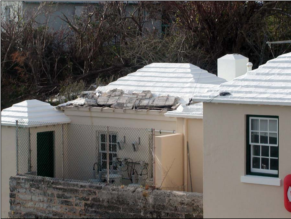
Figure 7. Leading-edge, "peel back", Swing Bridge St George's (south facing).
