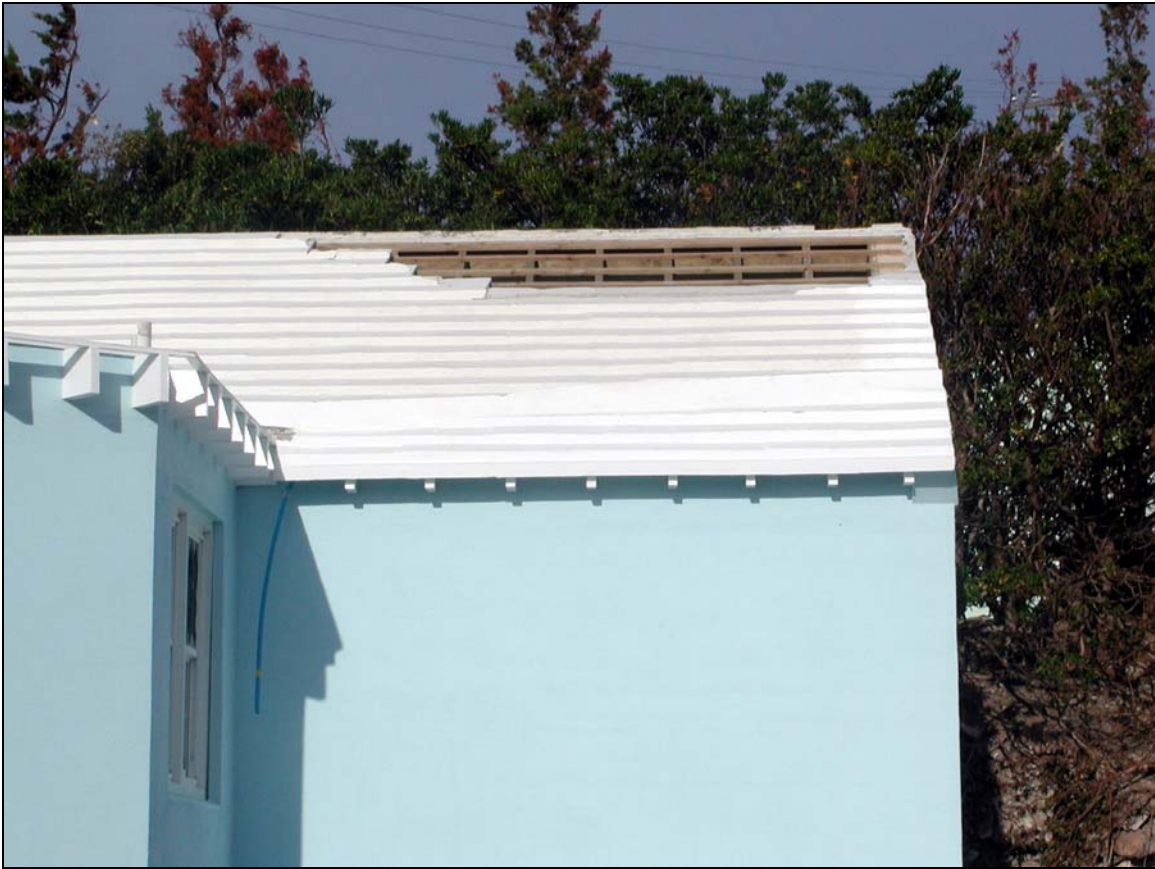
Figure 9. Roof crest damage, Wellington Lane St George's (west facing).
