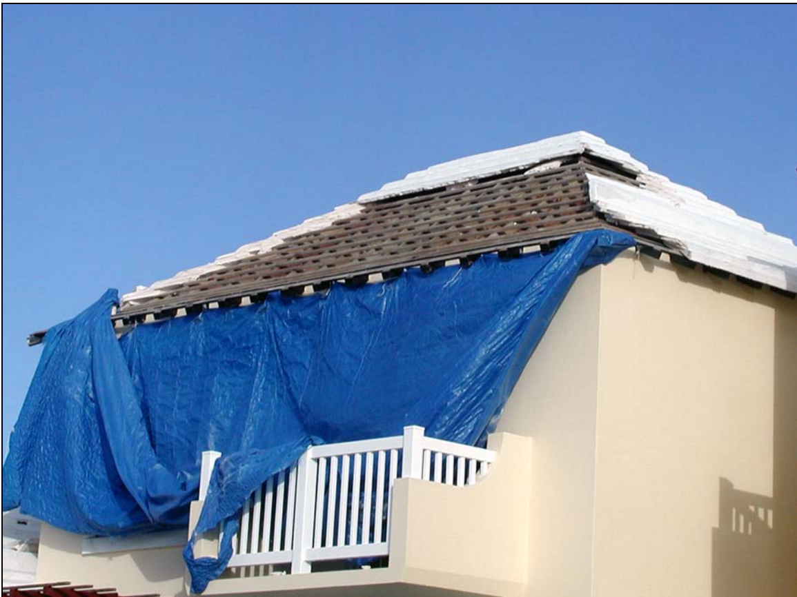
Figure 4. Less typical, extensive slate loss on windward side. St George's Club (south facing).
