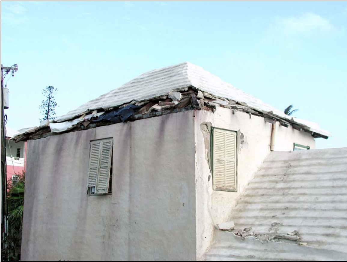
Figure 5. Historic house in St George's with exposed rafters (east and south facing).
